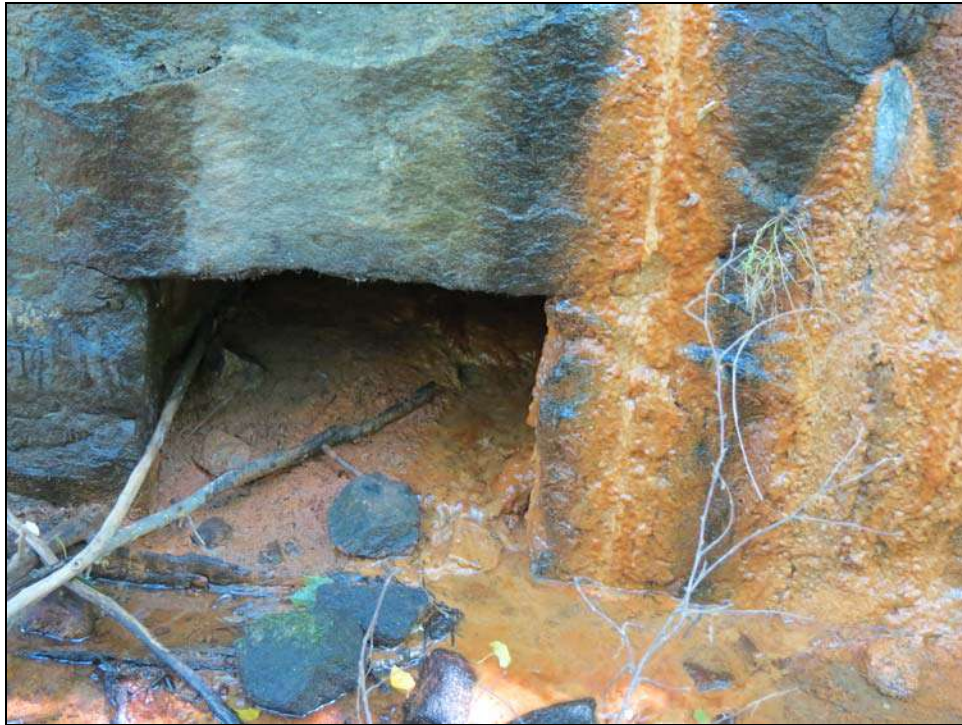
Figure 95. Architectural Resource WA1677 (Milburnie Dam), view of the east wall showing the drainage channel cut into the base of the wall.
