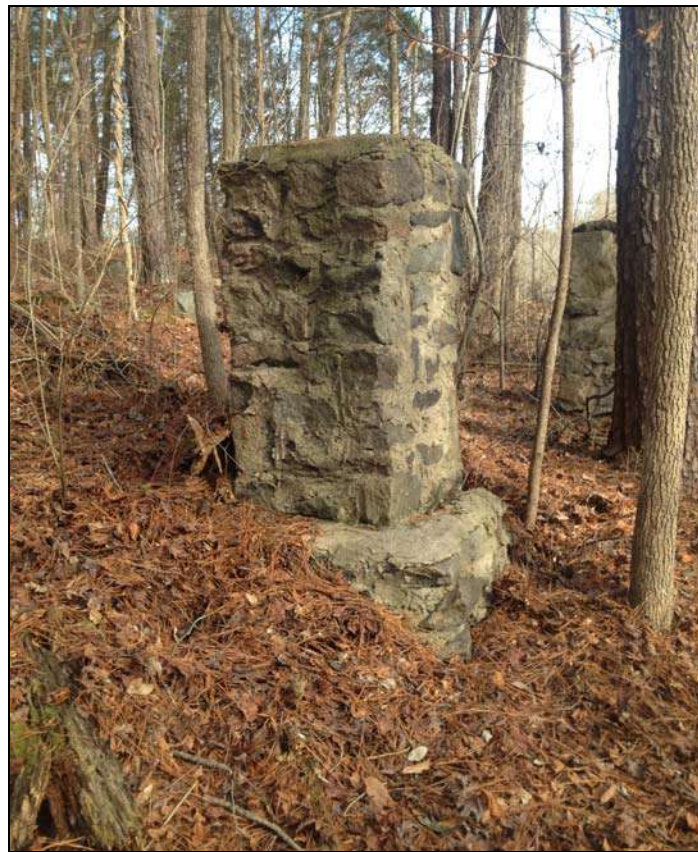
Figure 72. Site 31WA1872/1872** - Area 5, Structure 3 (close-up of stone pier foundations), view northwest.
