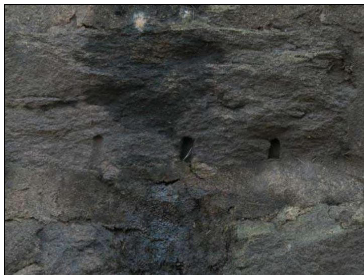
Figure 96. Architectural Resource WA1677 (Milburnie Dam), view of quarry marks in the east wall.
