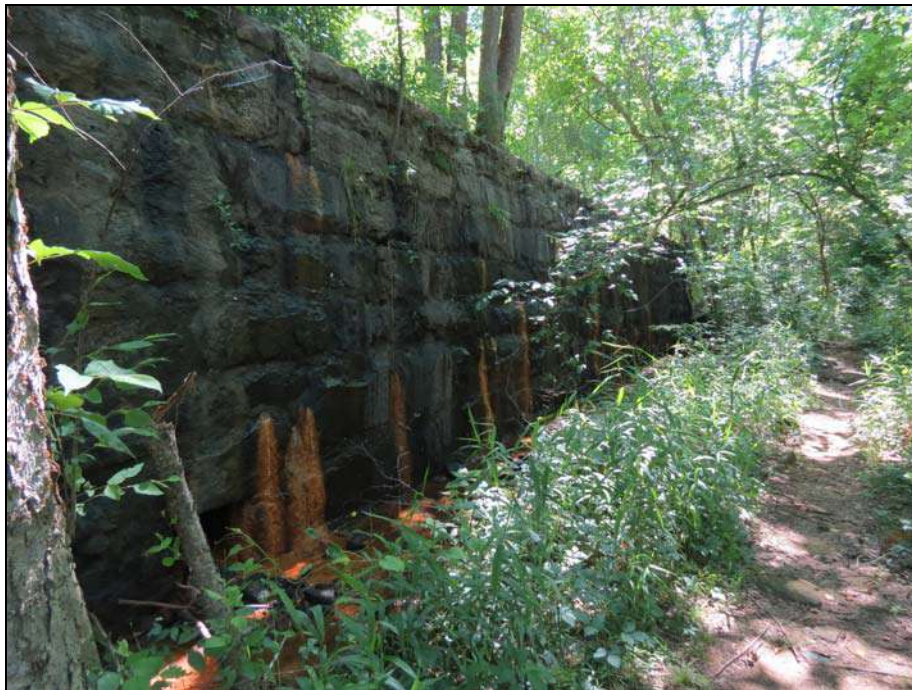
Figure 94. Architectural Resource WA1677 (Milburnie Dam), view of the east wall showing the drainage channel and granite blocks and pathway south of the dam, view east.
