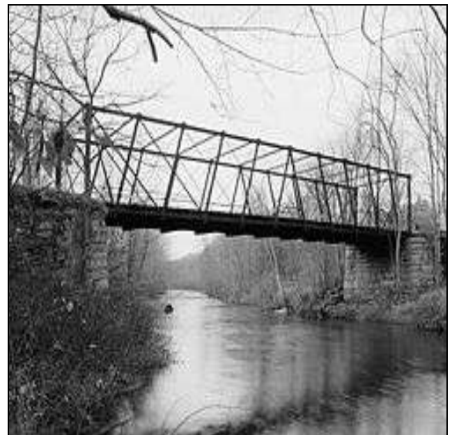
Figure 86. Post Patent Truss Bridge (Ponakin Bridge) example.
